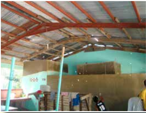
The white marks are where the sun is shining through holes in the roof.
