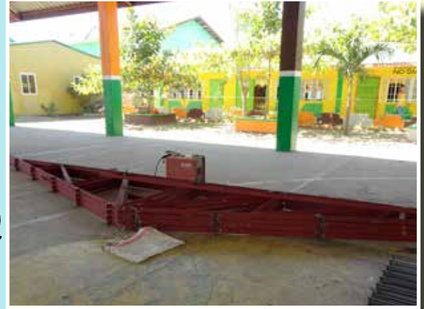
Window frames and roof supports all fabricated on site
