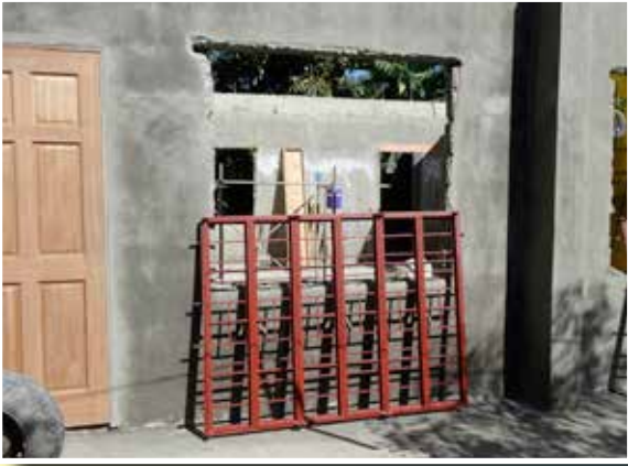
Window frames and roof supports all fabricated on site
